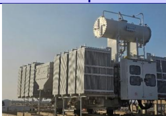
Inverter-Duty Transformer
